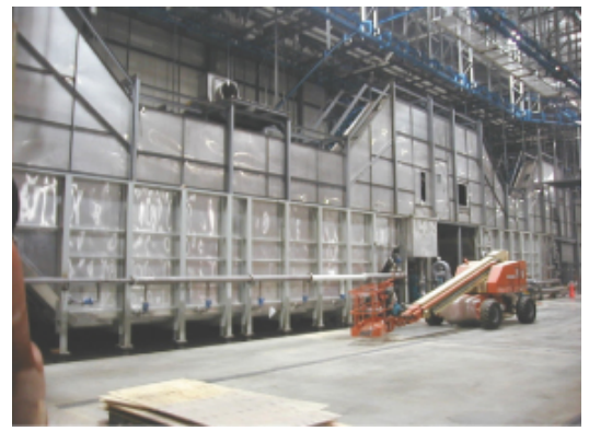
H.M. White Phosphate and E Coat Line Under Construction at an Automotive Plant
